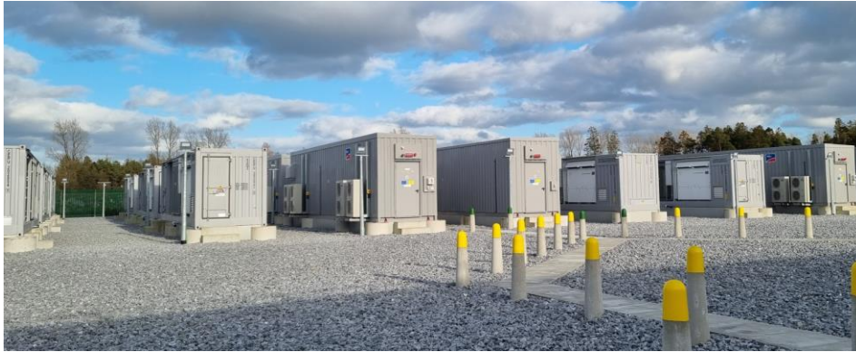
Figure 2.4 Image showing typical arrangement of LDES enclosures
